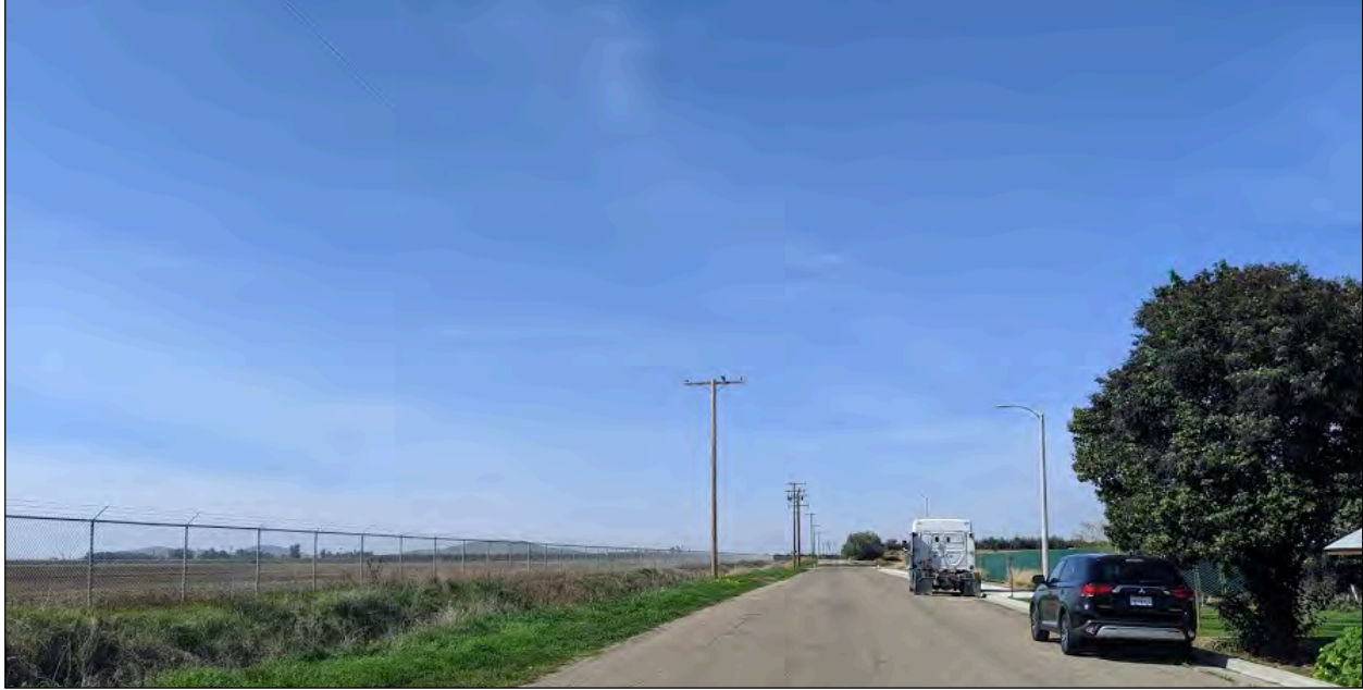
Figure 11. Photograph of the Project site, looking west, showing the alignment of the southern section of the new pipeline that will be installed under a paved road, surrounding residential development (right), and an existing detention basin (left).
