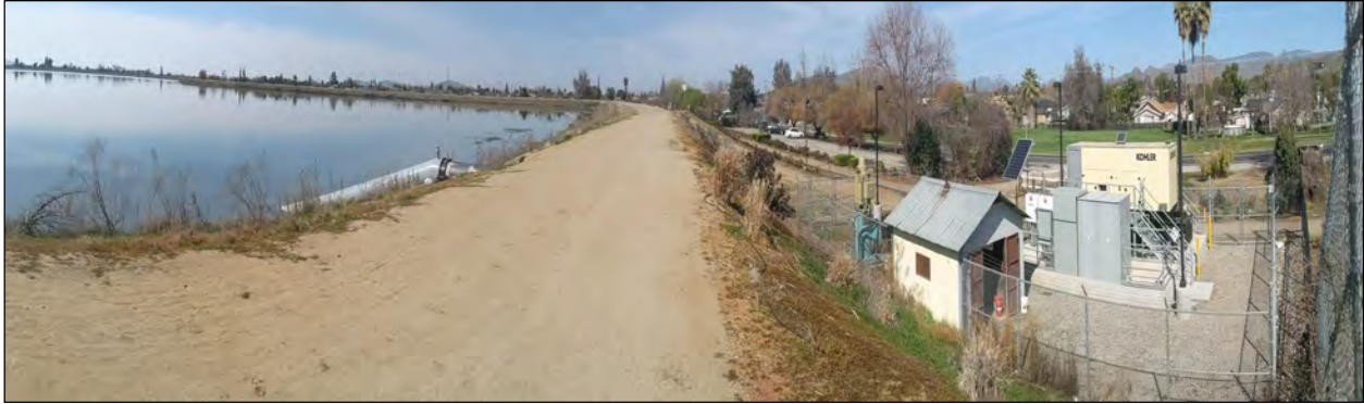
Figure 9. Panoramic photograph of the Project site, looking west, showing Bravo Lake (left), the alignment of the northern section of new pipeline that will be installed under a paved walking trail (right of levee), and Manzanillo Pump Station (right).
