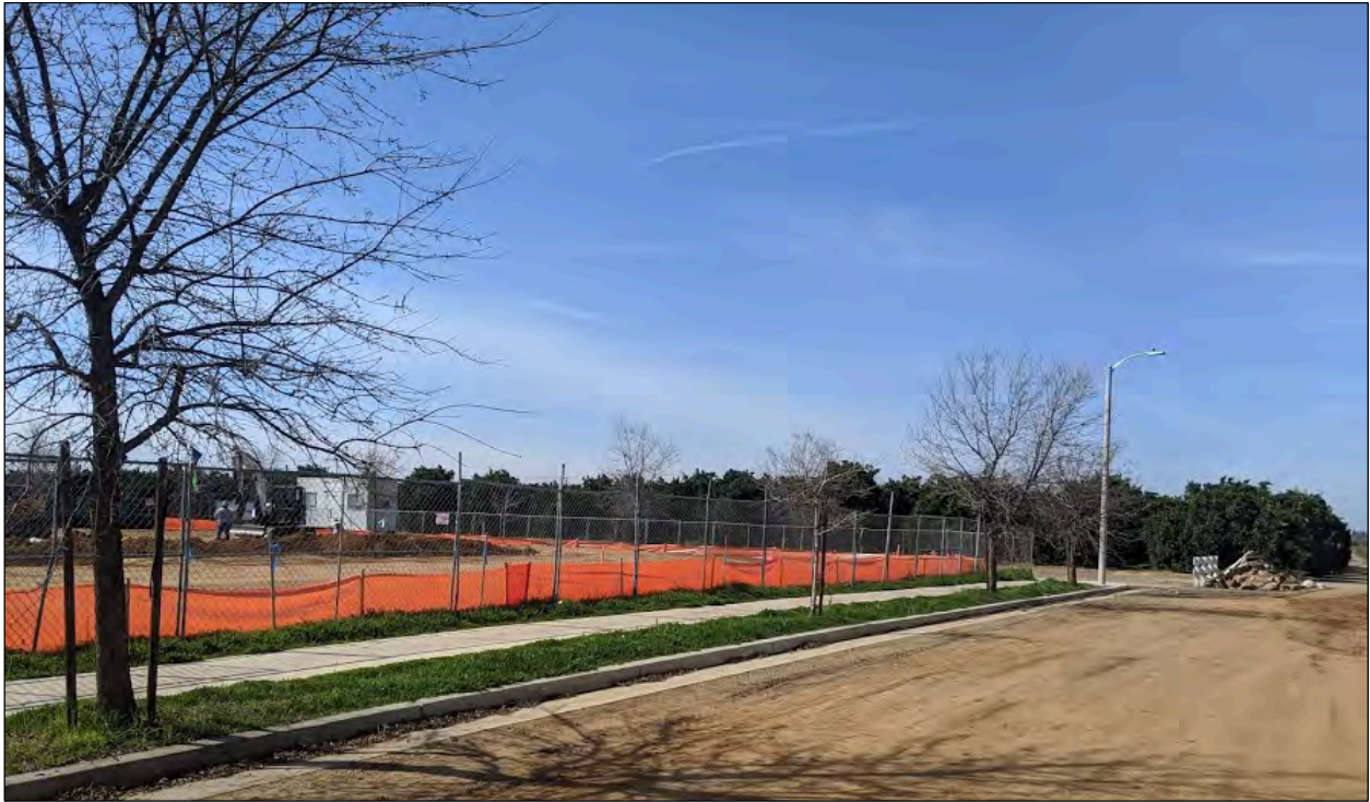
Figure 7. Photograph of the Project site, looking southwest, showing the alignment of the northern section of new pipeline that will be installed under a dirt road.
