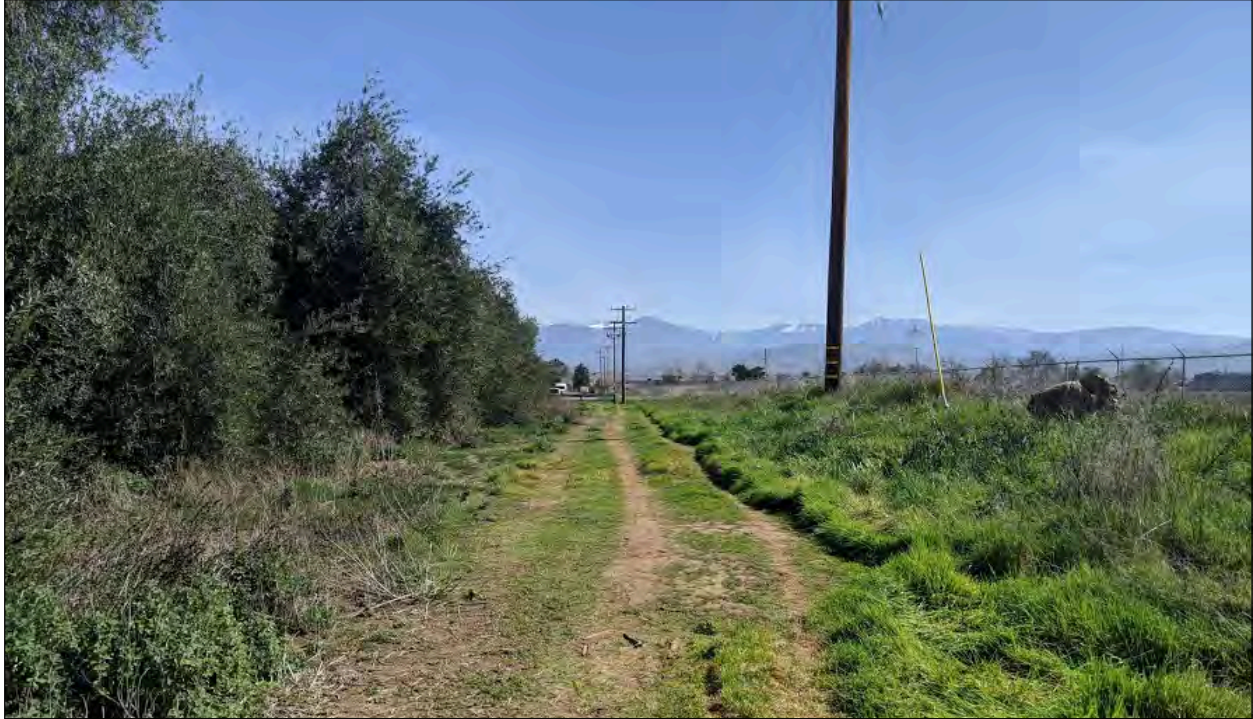
Figure 10. Photograph of the Project site, looking east, showing the alignment of the southern section of new pipeline that will be installed under a dirt road immediately east of the new stormwater basin.
